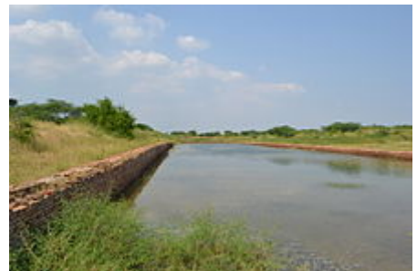
The dock, with a canal opening to allow water to flow into the river, thereby maintaining a stable water level.
