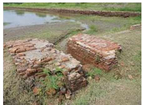
Remains of canal opening, built with burnt bricks.
